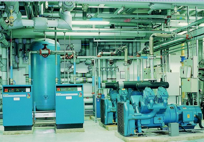
***The V-Compact is a free standing, single acting, lubricated or oil free unit set on anti-vibration mounts and is suitable for air or water cooling. Pressures range from 1.5 to 10.5 bar g, and power from 18 to 63 kW.***
